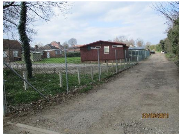
Fence along east boundary.
